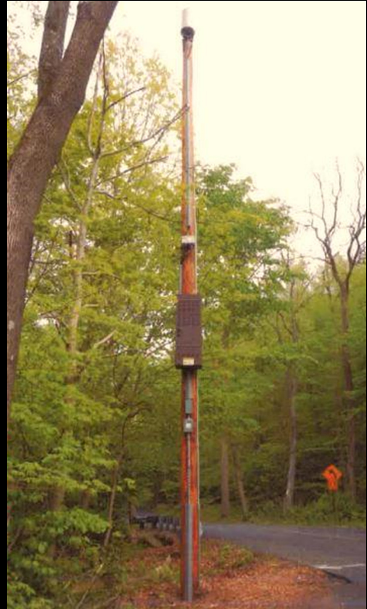
New Utility Pole
